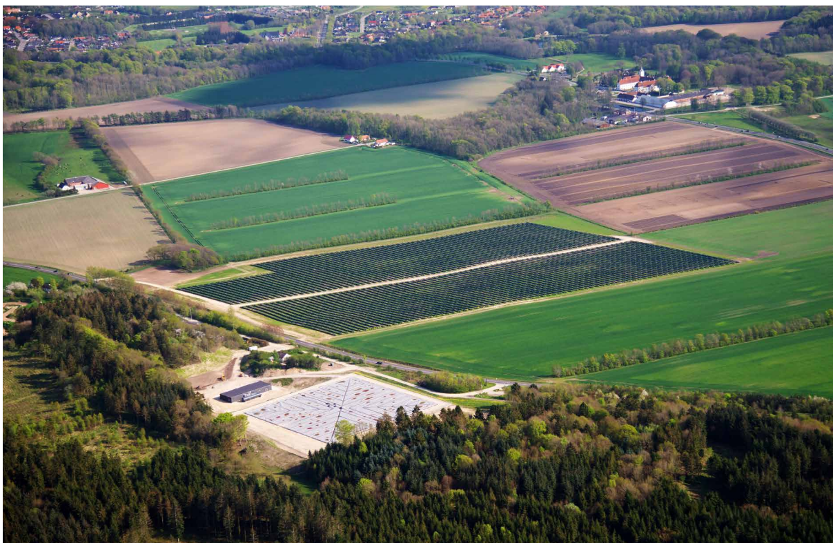
PTES and sun collector system in Dronninglund, Denmark. Source: NIRAS
