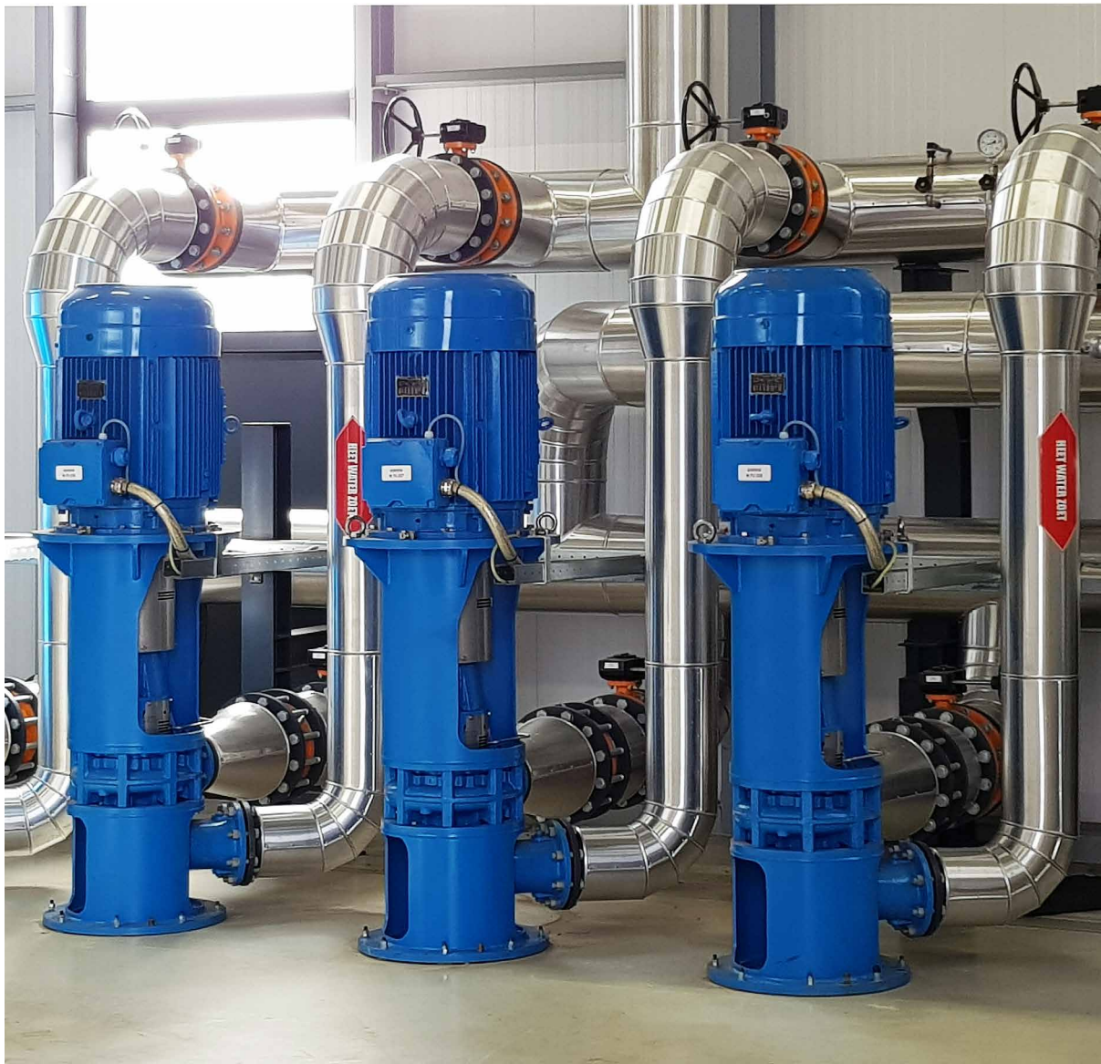
Surface facility equipment for the geothermal installation at Middenmeer, The Netherlands. Source ECW Energy
