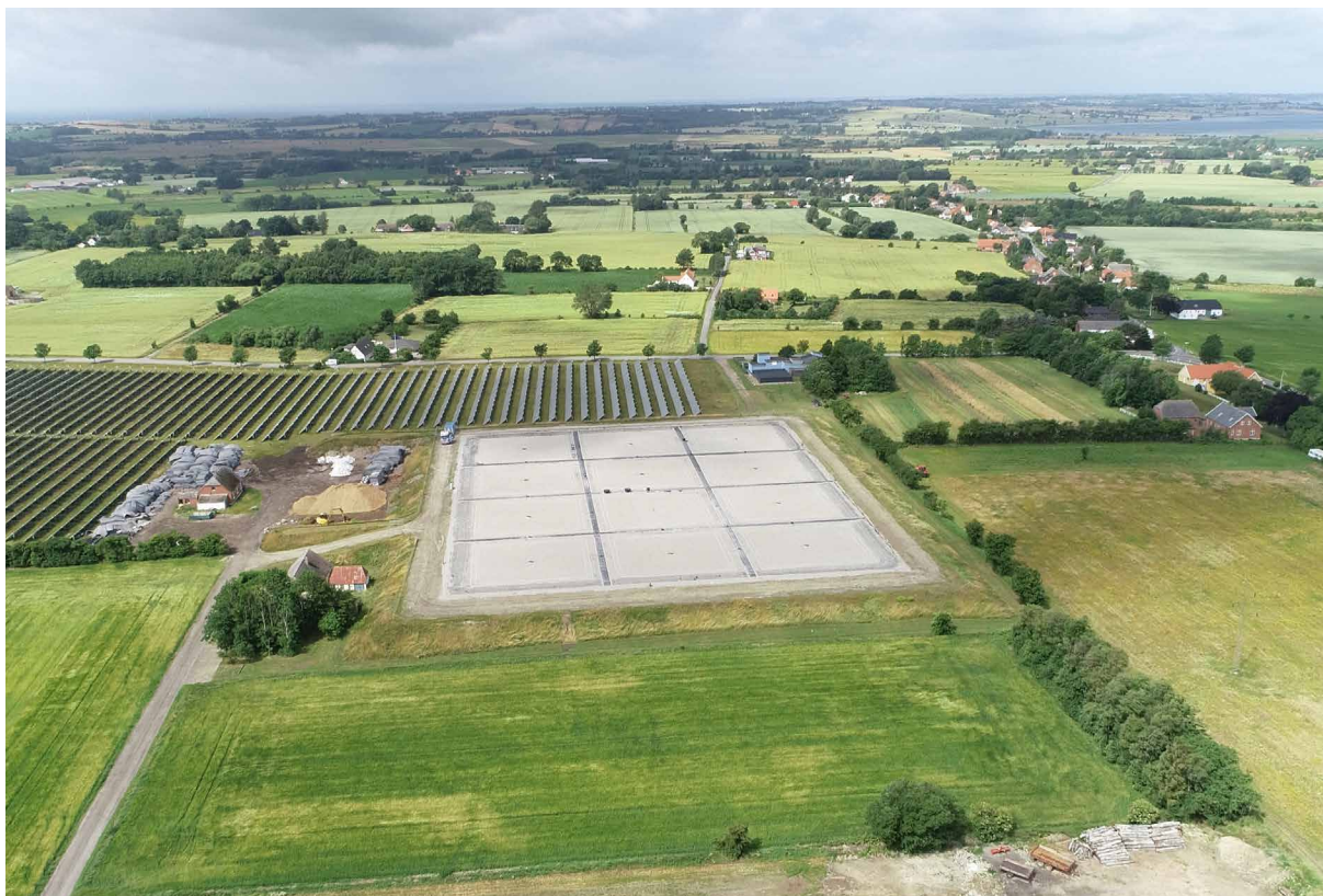
PTES and sun collector system in Marstal, Denmark. Source: Aalborg
