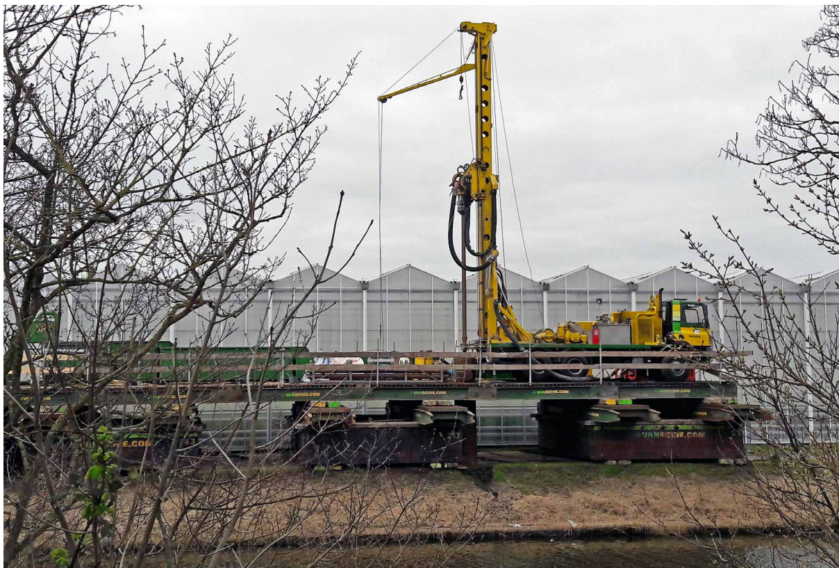
Drilling platform for HT-ATES in Middenmeer, The Netherlands. Source: ECW Energy
