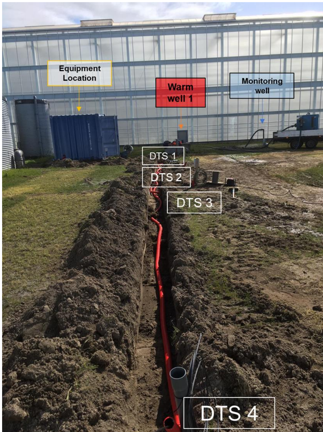
Figure 6: Overview of the monitoring facilities around ‘warm well 1’. New locations (Sept 2019) are: DTS 2 (deep), DTS 3 (deep) and the monitoring well. (When compared to figure 4, the viewpoint is from right to left).
