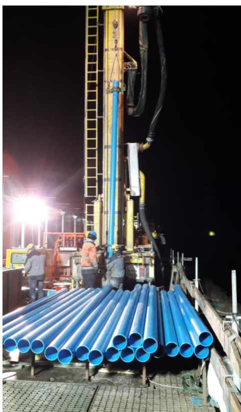
Figure 7: Drilling the test well at the Dutch demonstration site.
